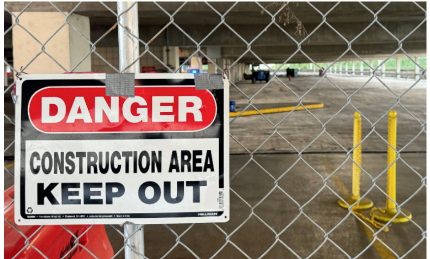
Blocked-off construction areas in Parking Garage A. NOAH SCHLARMAN
